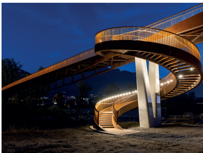
LaneLED WALL, Passerelle de Torretta Bellinzona
